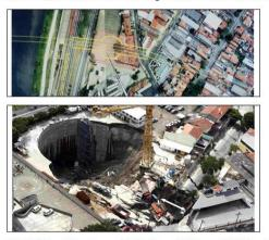
Eigure 1. The <u>Binheiros</u> station cavern and shaft collapse of 12<sup>n</sup> January 2007. The white arrow indicates the axis of the station cavern, and the fallen white car indicates the rear discontinuity.
